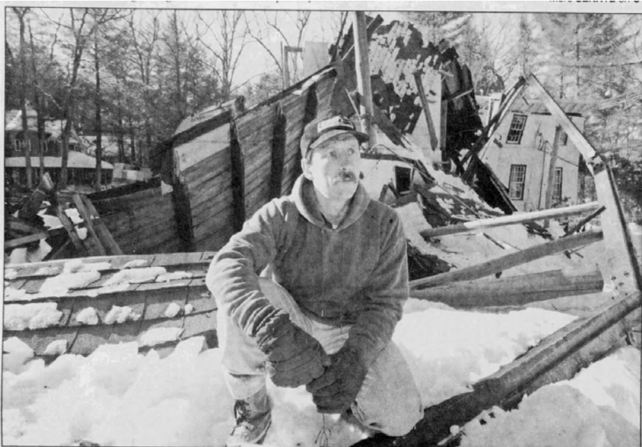
Bill Care, public works supervisor for Mount Gretna Borough, takes a break from salvage operations at the Chautauqua Playhouse.
