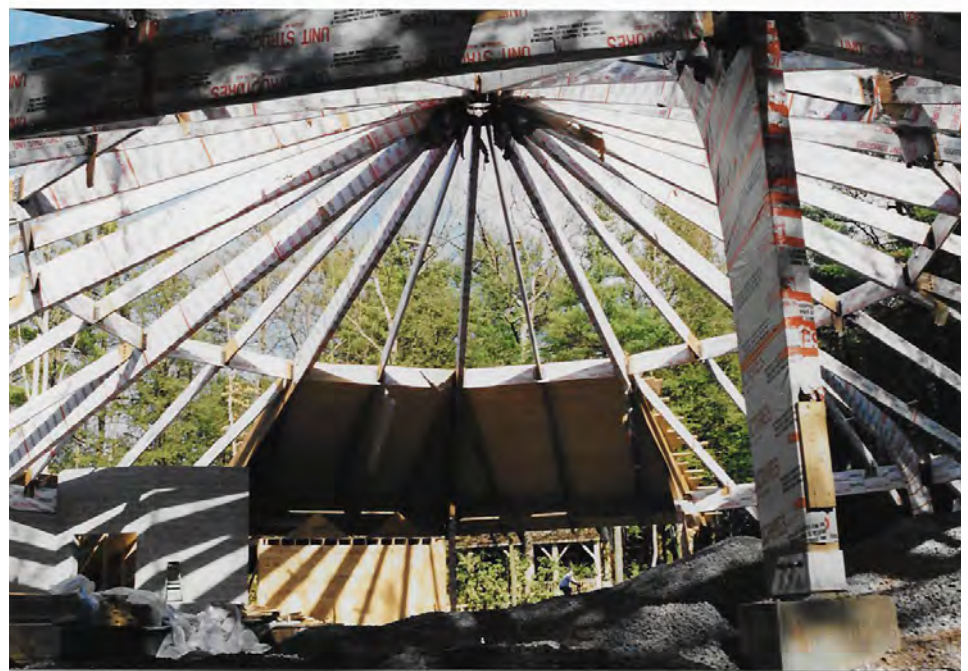
Above: The new Playhouse trusses as they went up in March 1995.
